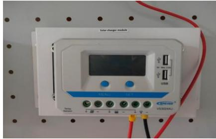
Gambar 2 Solar Charge Controller 30A 12V/24V Pwm
